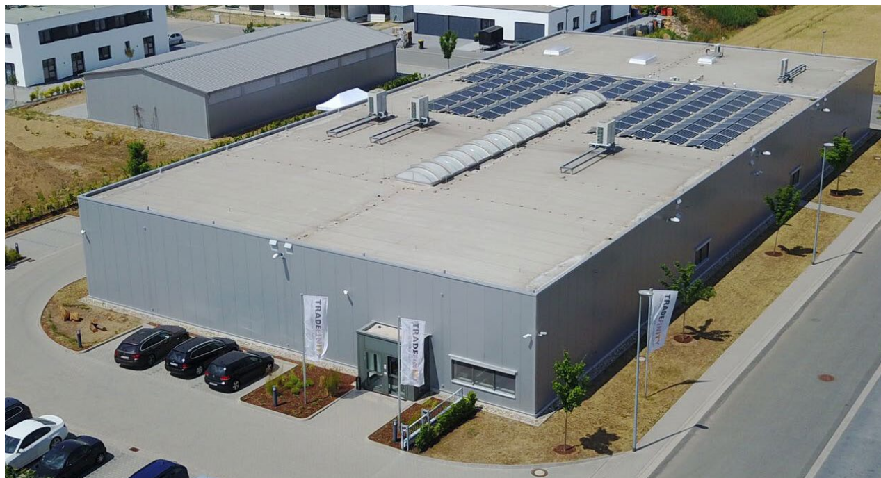
EPC's facility in Frankfurt, Germany
